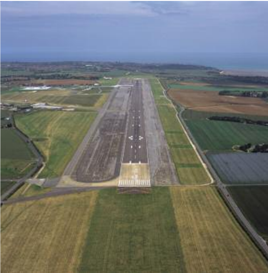
Situated just 60 miles east of London, Manston Airport's runway is 2,752 metres long x 61 metres wide.
